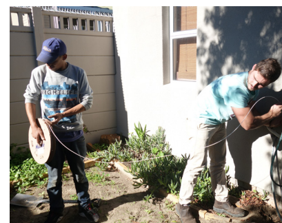
▲ Hand-pushable Miniflex removes the need for expensive blowing equipment
