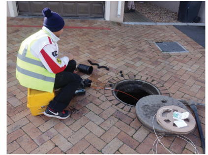
▲ Frogfoot installer deploying FTTH Miniflex through the drains
